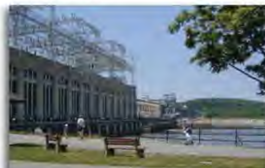
Conowingo Dam - Present Day
