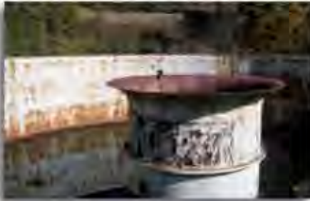
Surge Tank Tower - ROV Insertion
