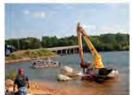
Excavator being towed out of water.
