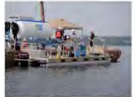
Barge with dive chamber & equipment setup.
